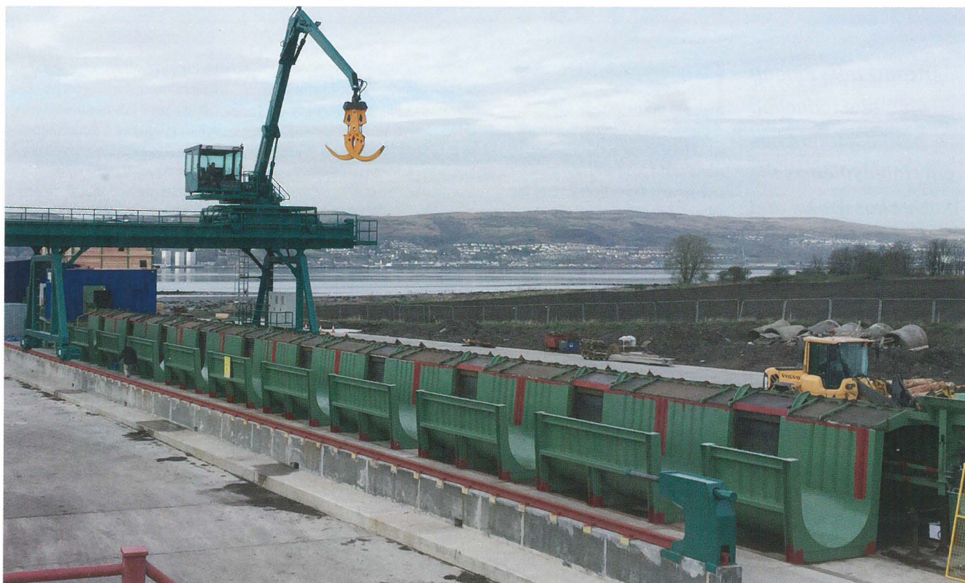
The log yard is 120 m by 55 m in size
